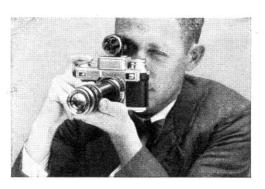
Since the centre of gravity lies in the lens when using a long-focus lens, it is desirable to hold the camera for exposure by grasping the lens with the left hand. This hand will then attend to the focusing, while the right hand steadies the camera and operates the shutter. The special finders for long-focus lenses are placed in the finder shoe on top of the camera, since the distance meter view-finder is not equipped with masks.
